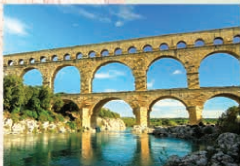
The first-century Pont du Gard aqueduct was built with 55,550 tons of soft limestone blocks.
